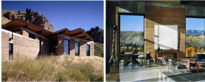
Left, TK pad residence exterior; right, TK pad living area showcasing distinctive EarthWall construction, photo courtesy Ward + Blake Architects.
